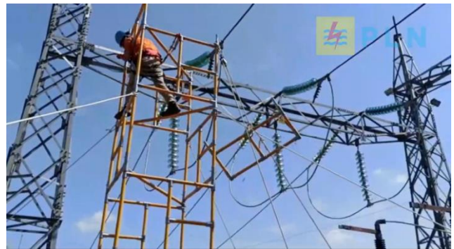
Fig. 1. Physical practice of scaffolding assembly and disassembly.
