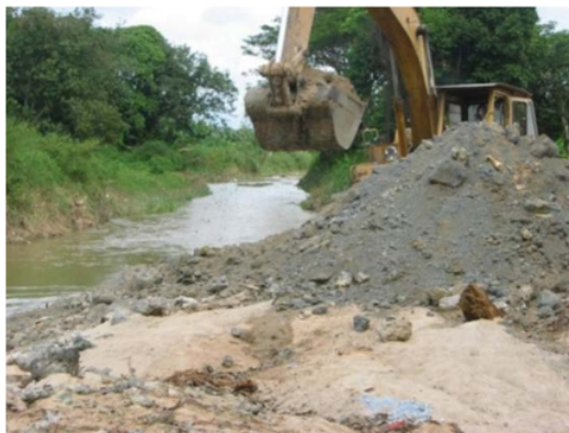
Fig. 1. Removing wastewater sludge from the river [15].
